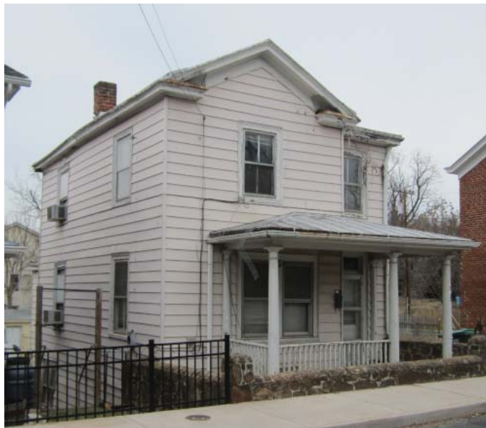
Traditional 2-over-2 house in Fifeville prior to demolition.
