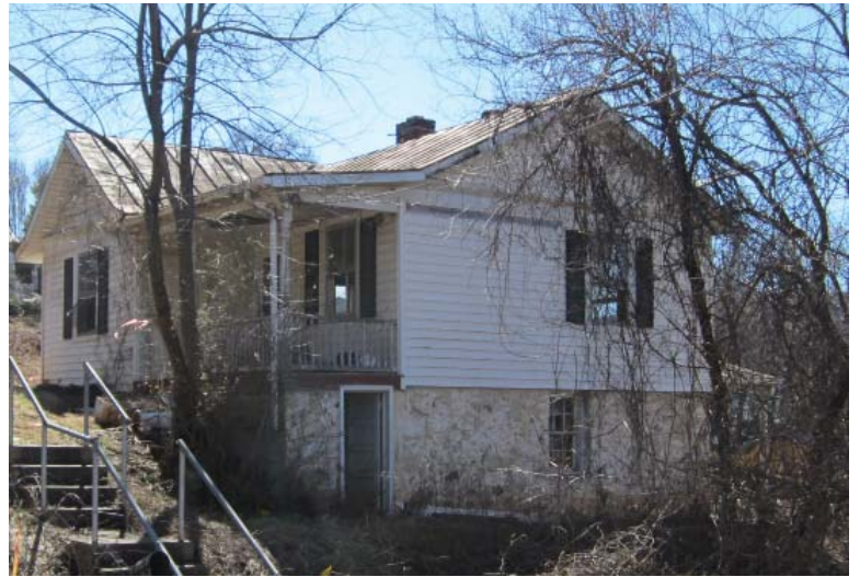
Unique house in Belmont prior to demolition.
